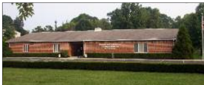
PASR Headquarters • Mechanicsburg, Pennsylvania
